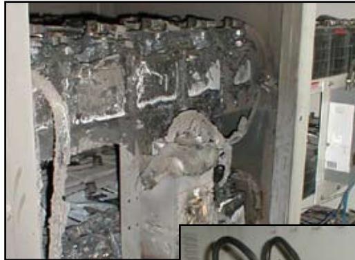
Thermal runaway effects on adjacent battery cabinet
