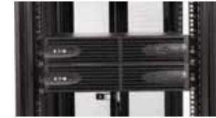
The Eaton 5130 UPS occupies 2U of rack space and the optional extended battery module also occupies 2U.
